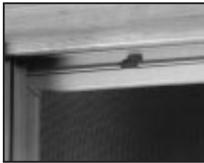
Proper seating of screen at head.
