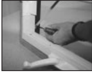
Releasing stud clip on awning hinge arm.
