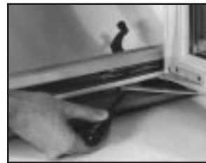
Releasing stud clip on hinge arm.
