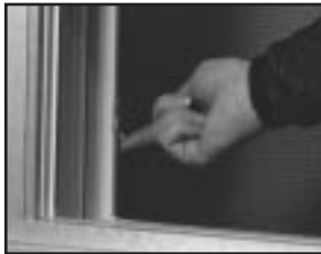
Lifting butterfly catch on screen.
