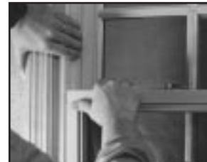
Pulling sash away from the jamb liner.
