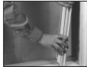
Slowly pull the bottom edge of jamb liner across sill and remove.
