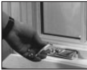
Removing the crank handle.
