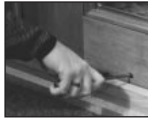
Adjusting the door rollers.
