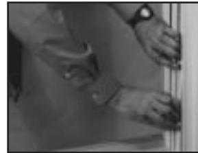
Compressing and disengaging jamb liner from frame.
