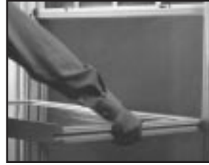
Removing the sash.
