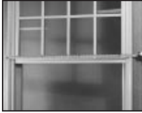
Making sure the frame is square. Check horizontal, vertical and diagonal measurements.
