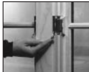
Lifting the sash lock lever.
