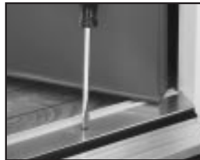
Adjustable, weathertight threshold.
