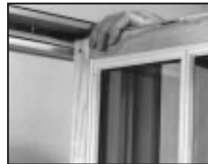
Removing sash - slide sash to end of hinge track.
