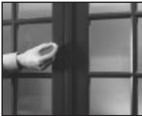
Use touch-up paint sparingly to cover small nicks or scratches.
