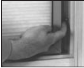
Loosen clips on System 2 storm panel.
