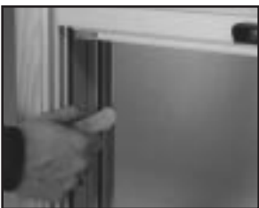
Lubricating the jamb liner with paraffin.
