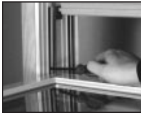
Adjusting the tension of sash shoe.
