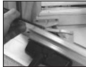
Releasing casement operator stud clip.
